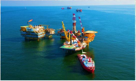
HYSY901/902 is self-elevating jack-up accommodation rig, designed to operate in water depths ranging from 5 meters to 35 meters.
